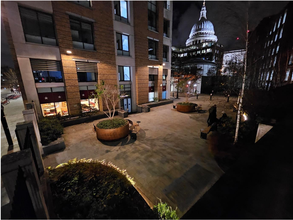
Phase 2 | Completed Off-Site Garden at night looking north from Nicholas Cole Abbey Church
