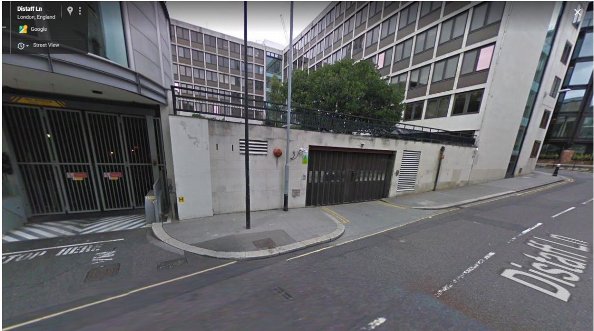
On-site Garden site and mastic asphalt footways | Before
